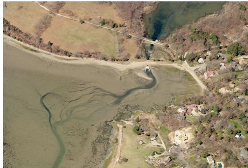
Culvert at CB-02b
